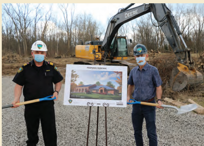
Breaking Ground with Fire Chief Ed Melanson and Mayor Wayne Redekop at the new Fire Station 4 location.
