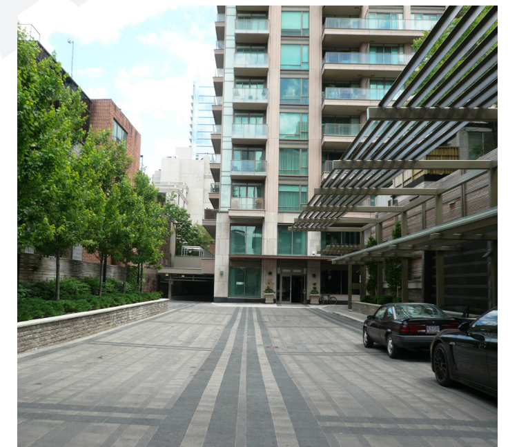
Figure 76: Example of a two-way laneway configuration that provides servicing and loading adjacent to buildings.
