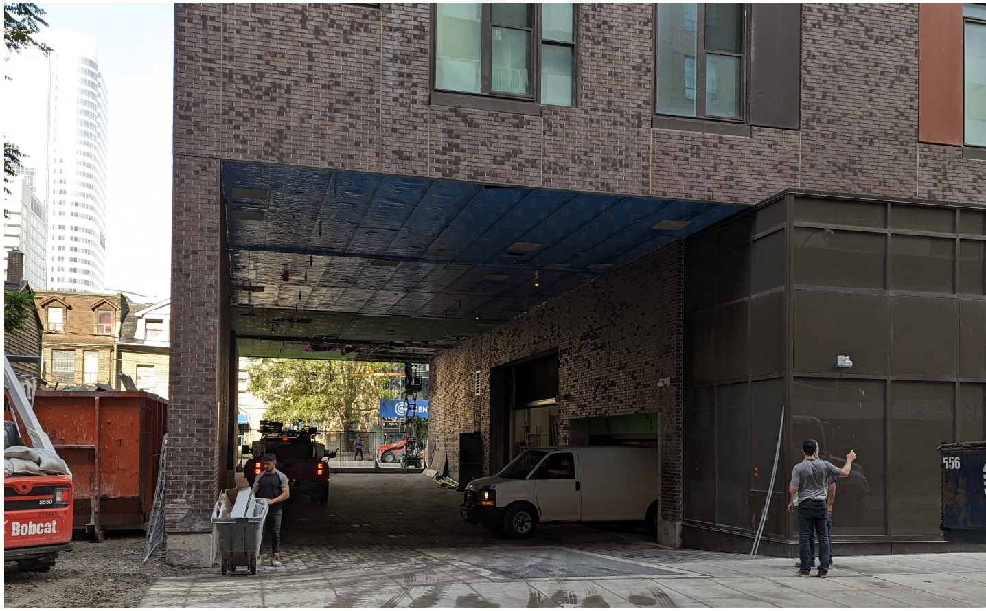
Figure 144: Waste collection areas should have an overhead clearance of 4.4 metres to ensure collection vehicle access is achievable.
