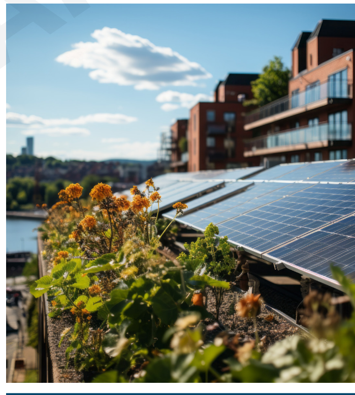
Figure 149: Green roof elements or community gardening efforts can be complemented by photovoltaic arrays.
