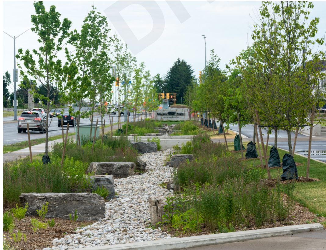
Figure 15: Bioswales located at walkways and parking lots can collect stormwater runoff to minimize the dependency on stormwater sewers.
