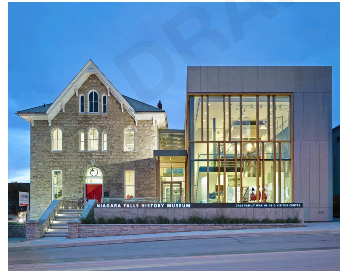
Figure 110: Additions should maintain a respectful relationship with heritage structures through the use of setbacks, the matching of datum lines, and visual breaks to ensure the dimensionality of the heritage building is legible (History Museum).
