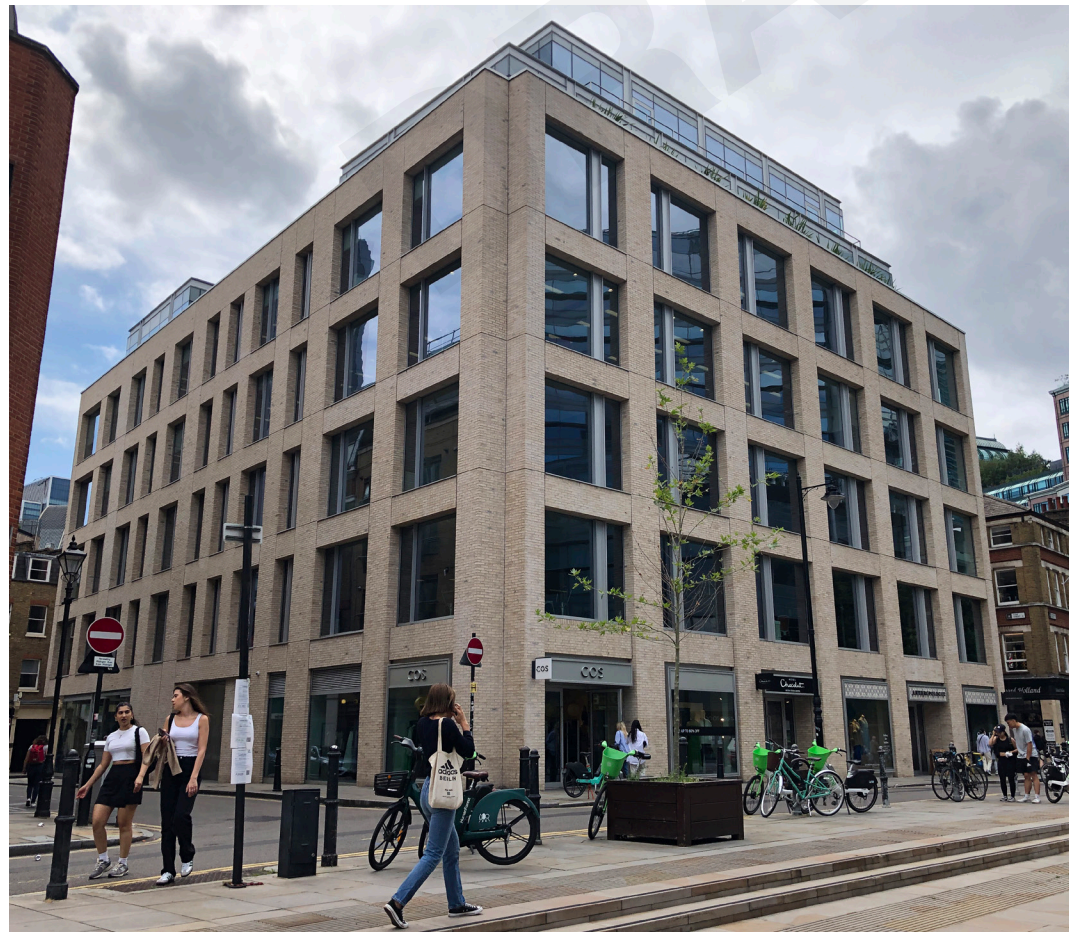
Figure 199: Mixed use buildings should promote ground floor transparency for retail or commercial units.
