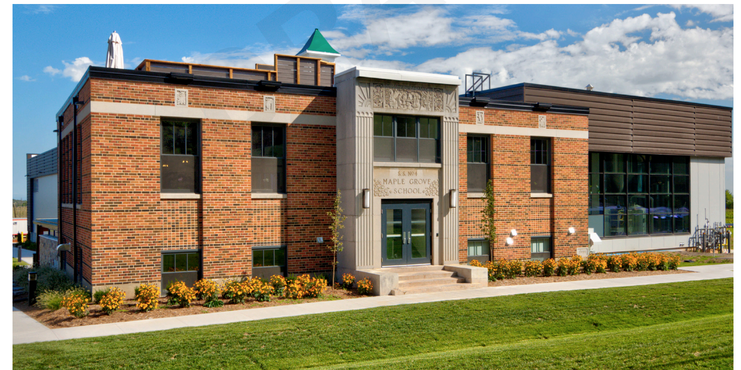
Figure 156: Ground floor elements should be retained and conserved (Bench Brewery)
