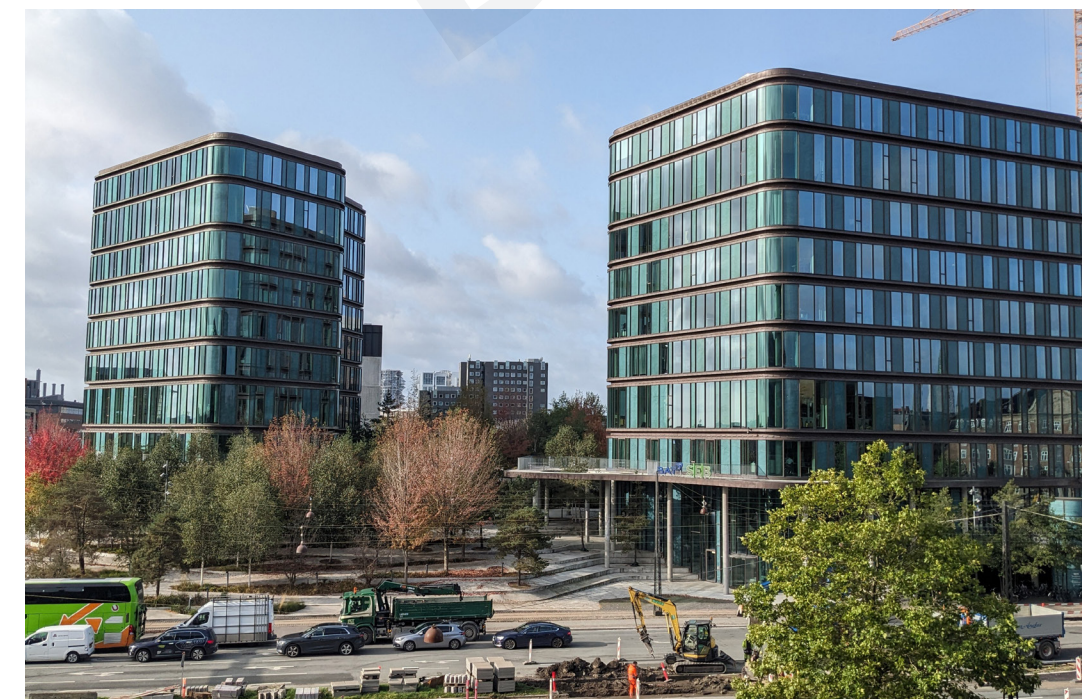
Figure 103: The relationship between buildings contributes to a comfortable site environment.
