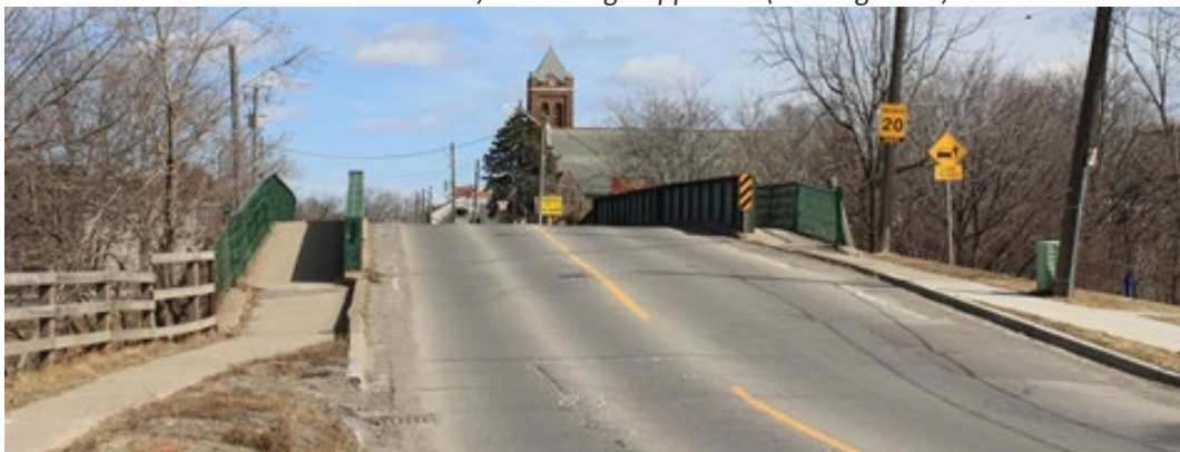
b) West Bridge Approach (Looking East)
