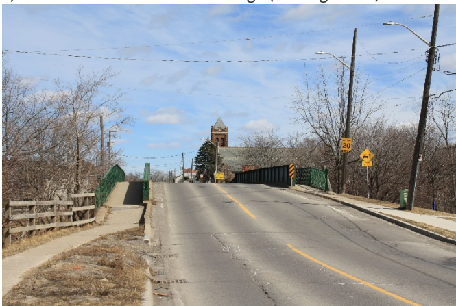
c) West Bridge Approach
