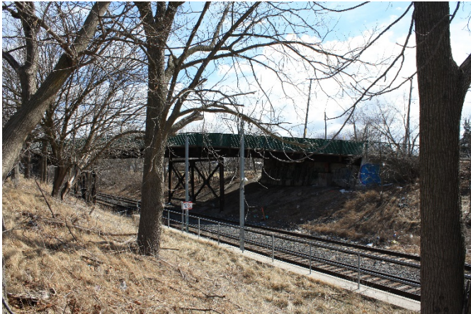
a) St. Paul Street West CNR Bridge (looking south)
