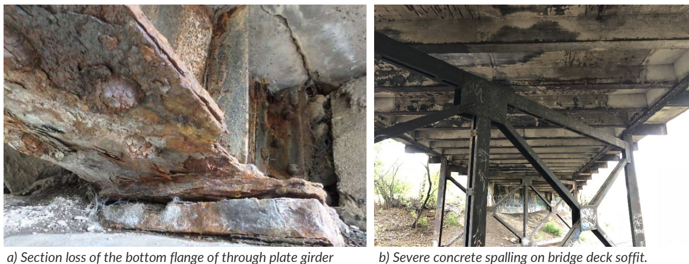
Figure 4-2: Existing Condition of Bridge Structure
