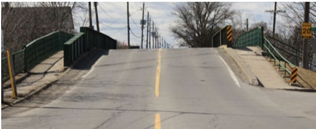
a) East Bridge Approach (Looking West)
