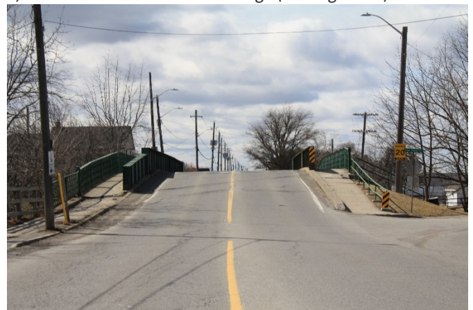
d) East Bridge Approach
