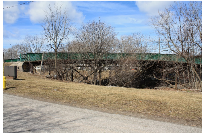
b) St. Paul Street West CNR Bridge (looking north)
