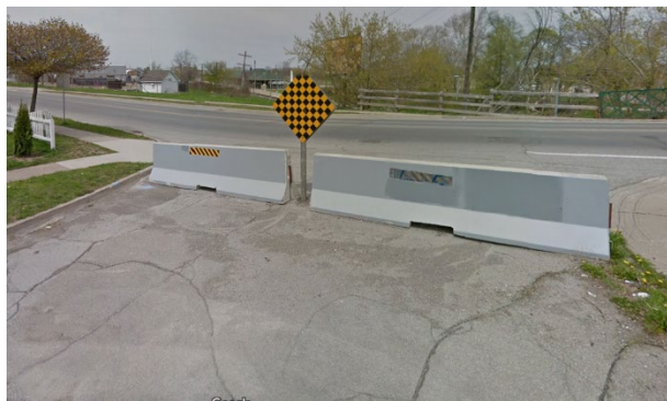
a) Leeper Street Temporary Closure
