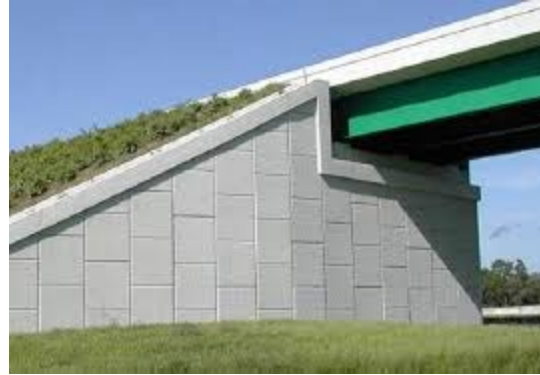
Figure 7-2: Typical Retaining Soil System (RSS) Wall Application
