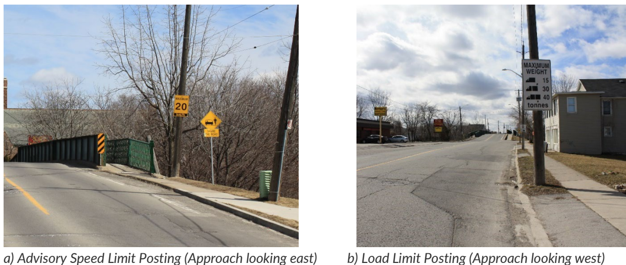
Figure 4-3: Triple Load Limit Posting (Approach Looking West)
