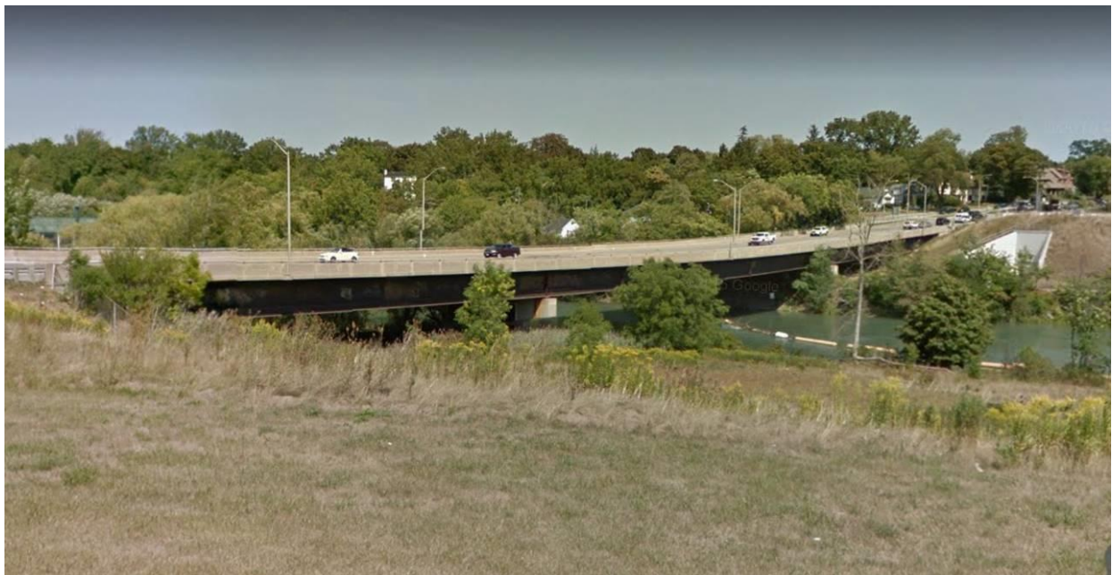
Figure 14: 12 Mile Creek Bridge, Fourth Avenue, St. Catharines, built in 1978 (Google Streetview)
