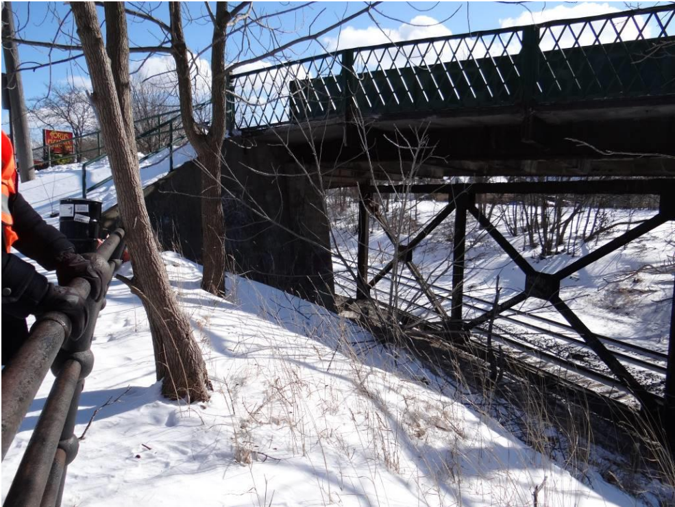
Plate 3: East portion of the north elevation including east abutment looking south.
