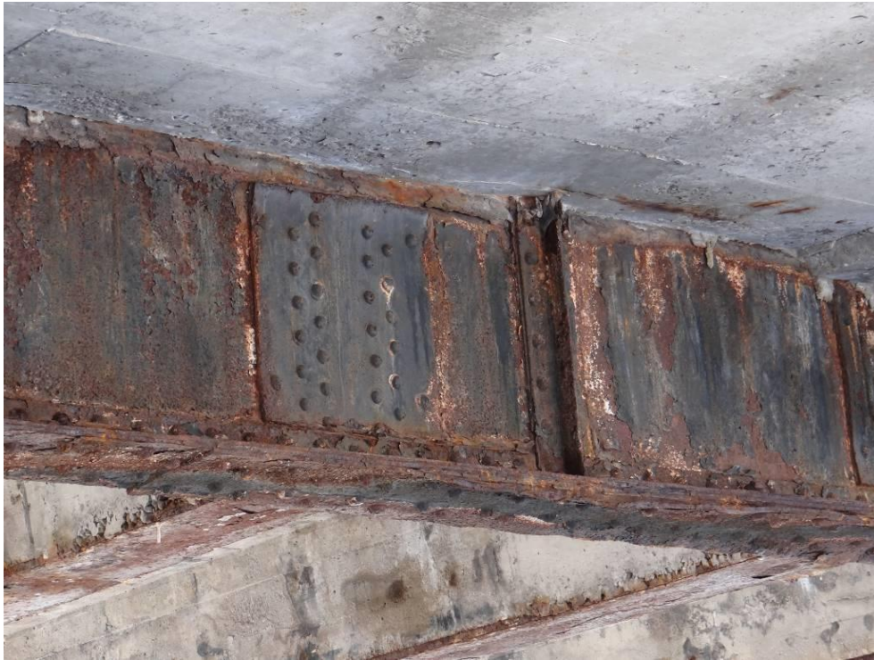
Plate 9: Riveted through-plate girder extending below the bridge deck.
