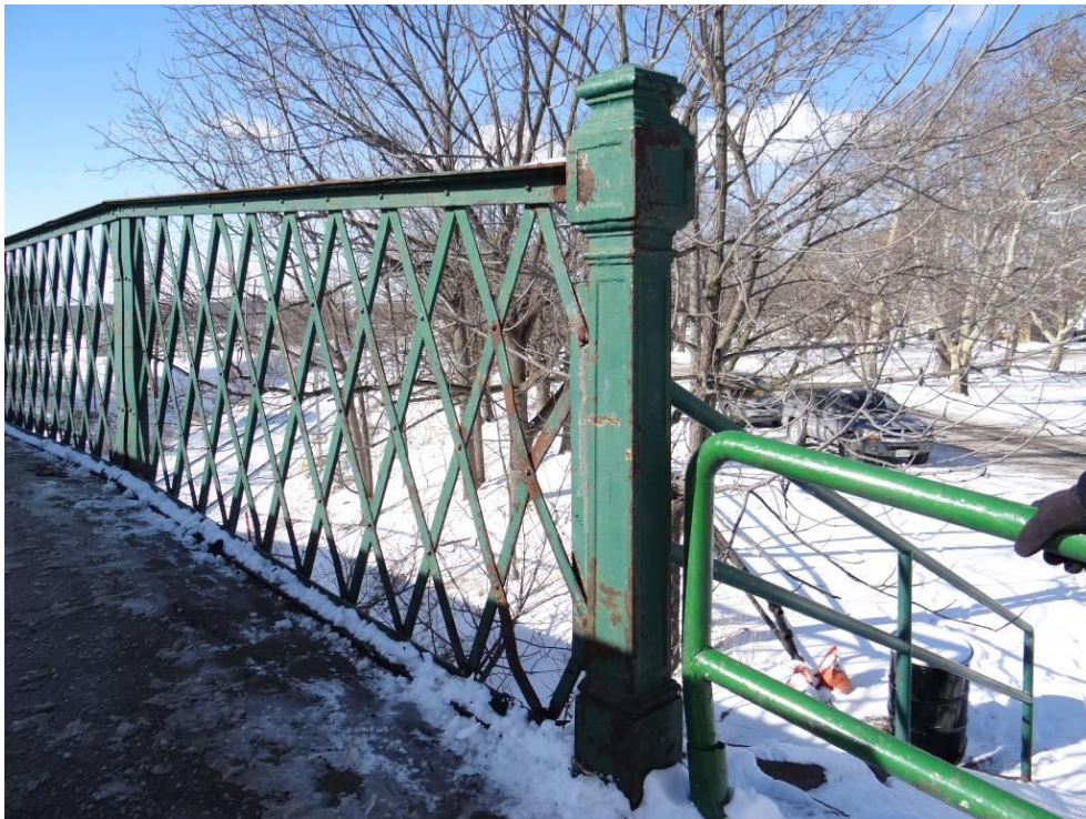
Plate 22: Steel lattice railing with steel newel post, looking northwest.
