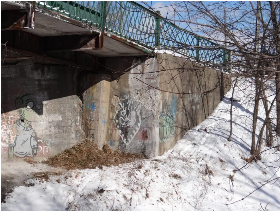
Plate 12: South and west faces of the east abutment, looking east.
