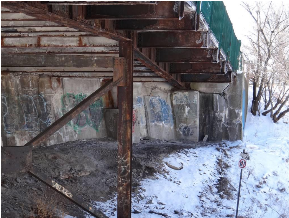
Plate 6: West abutment and transverse steel stringers, looking west.
