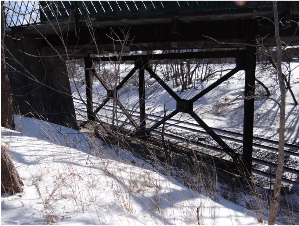
Plate 5: East bent, looking south.
