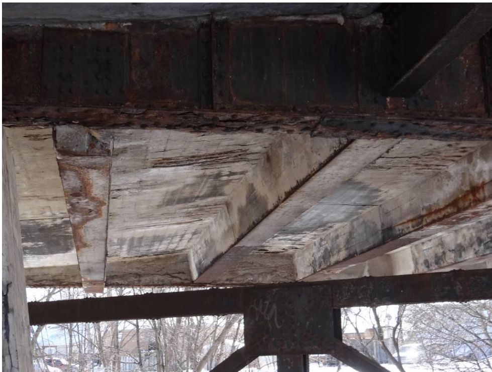
Plate 8: Bridge soffit showing transverse stringers and riveted through-plate girder, looking south.
