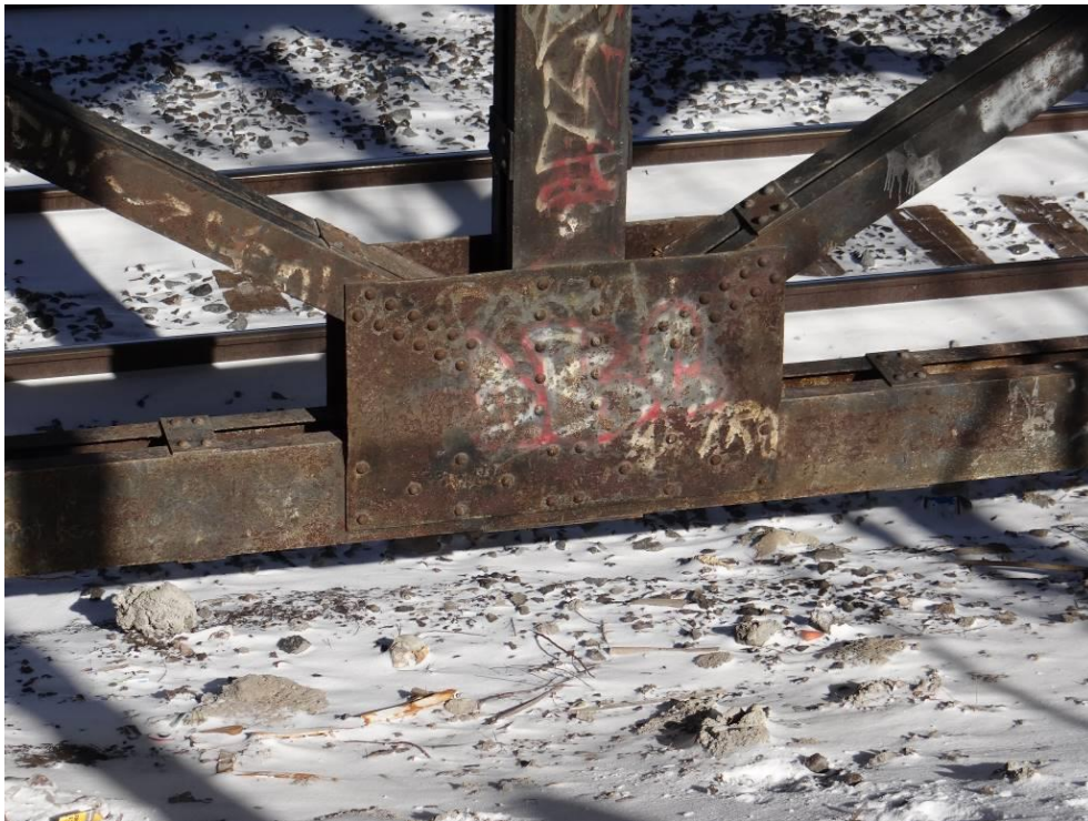
Plate 16: Detail of riveted connection on west bent, looking northeast.
