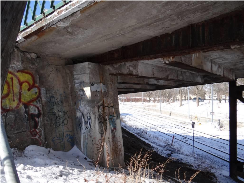
Plate 13: South face of the west abutment, looking north.
