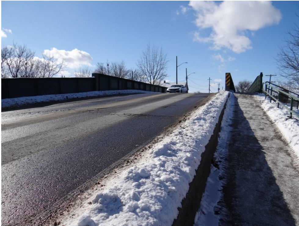
Plate 17: East span of the bridge at deck level, looking west. Note the steep slope of the approaches.
