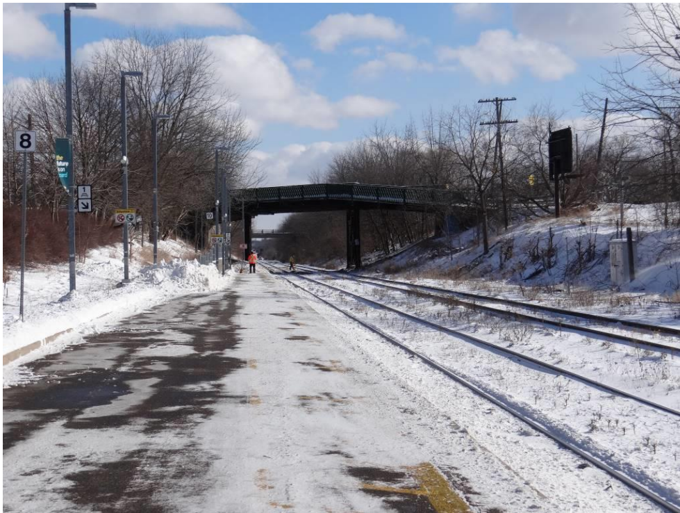
Plate 28: North elevation of the subject bridge, looking south from the platform of the St. Catharines Train Station.
