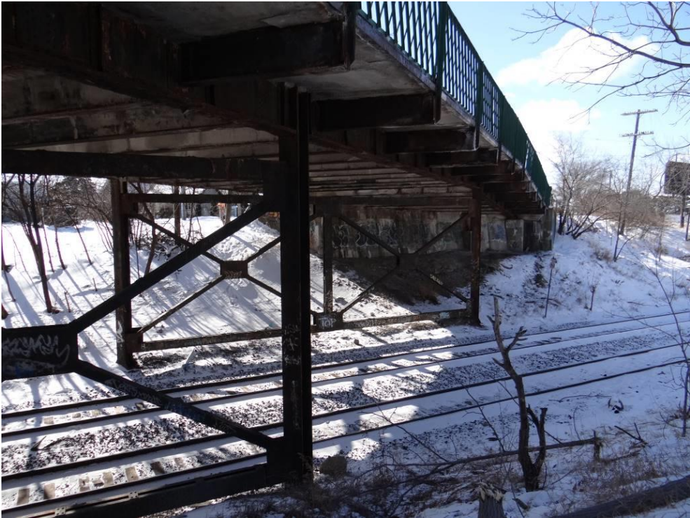
Plate 4: Substructure of the bridge, looking west from the east abutment.
