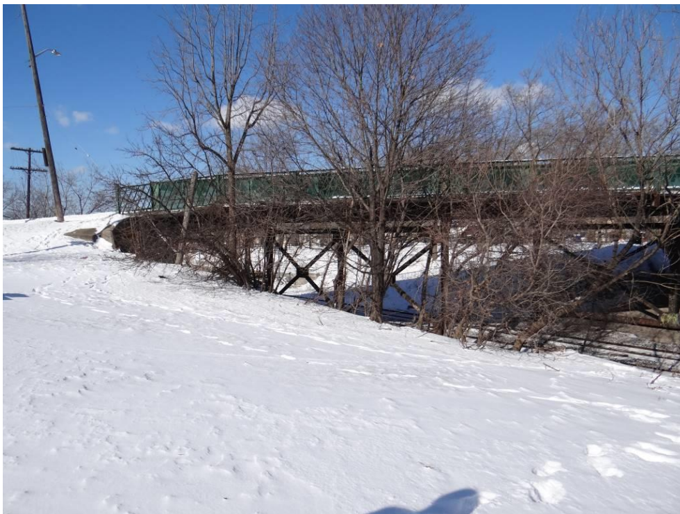
Plate 2: West portion of the south elevation, looking east.
