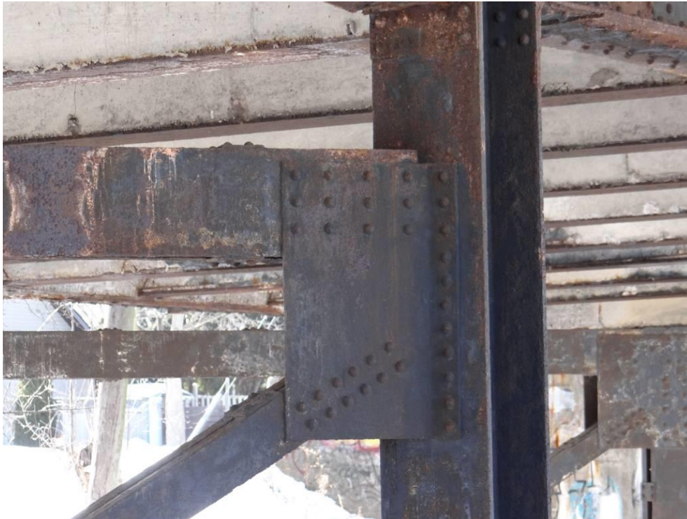
Plate 15: Detail of riveted connection on east bent, looking southwest.
