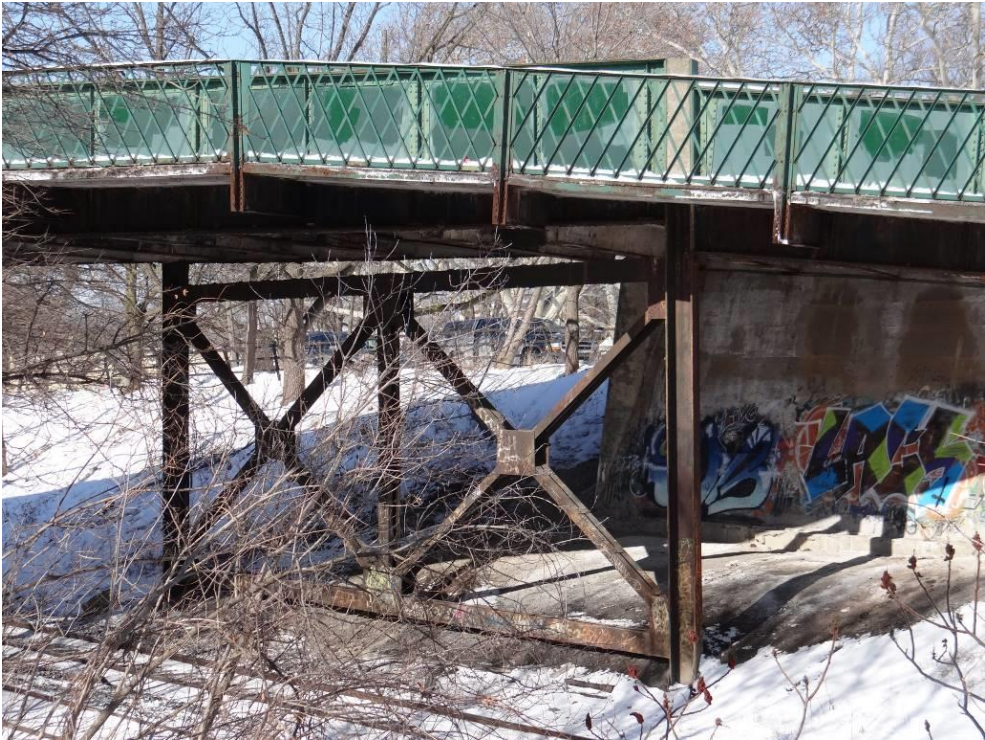
Plate 14: East bent, looking northeast.
