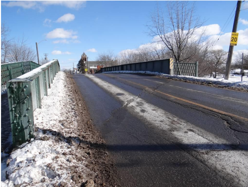
Plate 23: West bridge approach, looking east.
