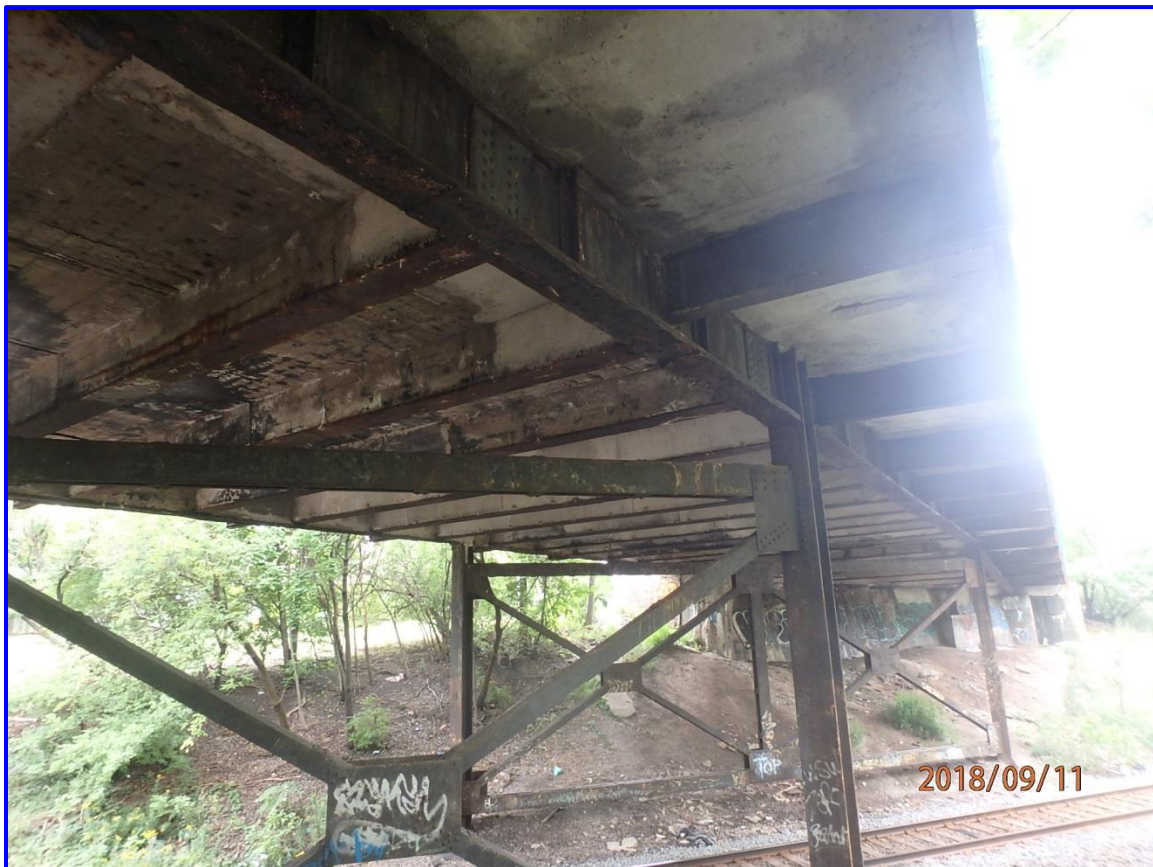
Photograph 4 – Underside of structure looking southwest
