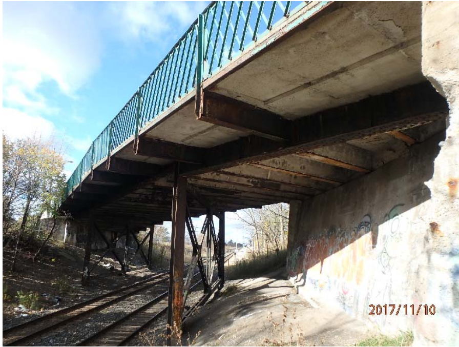
Photograph No. 1: 0530: South elevation
