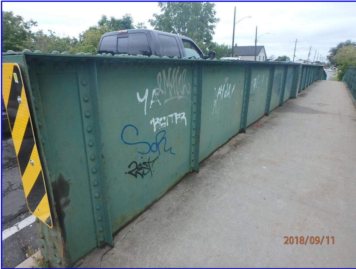
Photograph 1 – East end of the north through-plate girder
