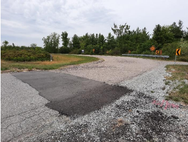
Plate 1: Lands beyond disturbed road ROW require Stage 2 survey
