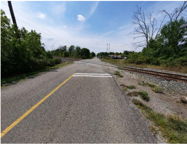
Plate 5: Disturbed road and rail ROW; no potential
