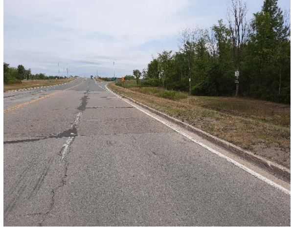
Plate 2: Lands beyond disturbed road ROW require Stage 2 survey
