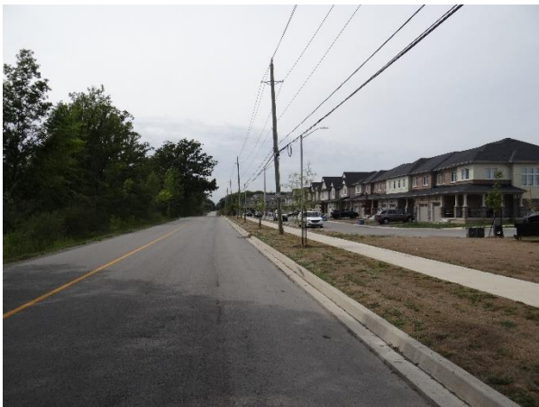
Plate 5: Residences on Brown Road, looking west
