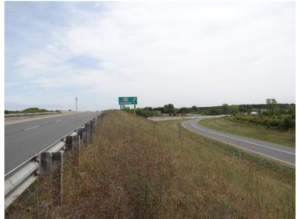
Plate 14: Lyons Creek interchange with the QEW, looking east.
