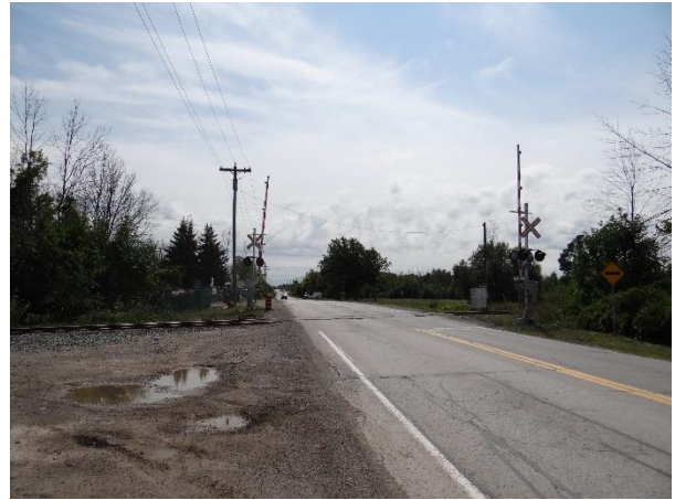
Plate 8: CPR tracks crossing Montrose Road, looking south.
