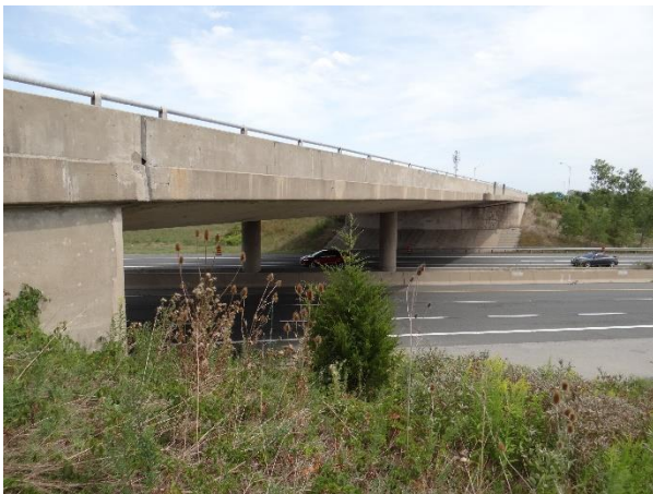
Plate 15: Lyons Creek Road bridge over the QEW, looking northeast.
