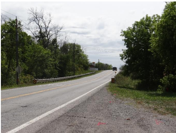
Plate 9: Looking south on Montrose Road from Grassy Brook Road.
