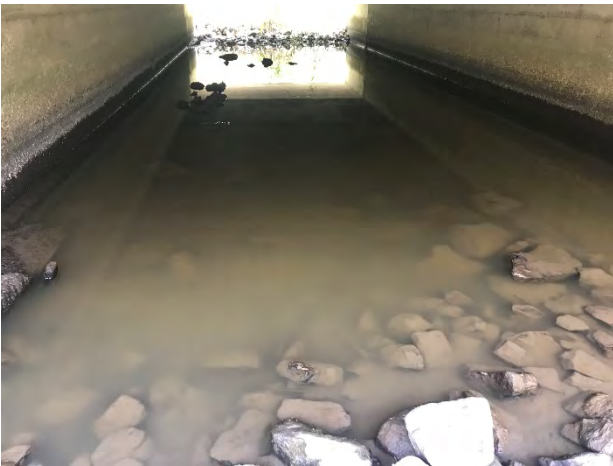
PHOTO 44 (LEFT): SCOUR PROTECTION AT INLET AND PONDED WATER WITHIN CULVERT STRUCTURE.
