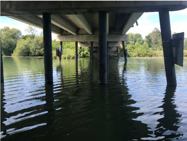
PHOTO 27 (LEFT): VIEW UNDER EXISTING BRIDGE LOOKING NORTH FROM SOUTH BANK.
