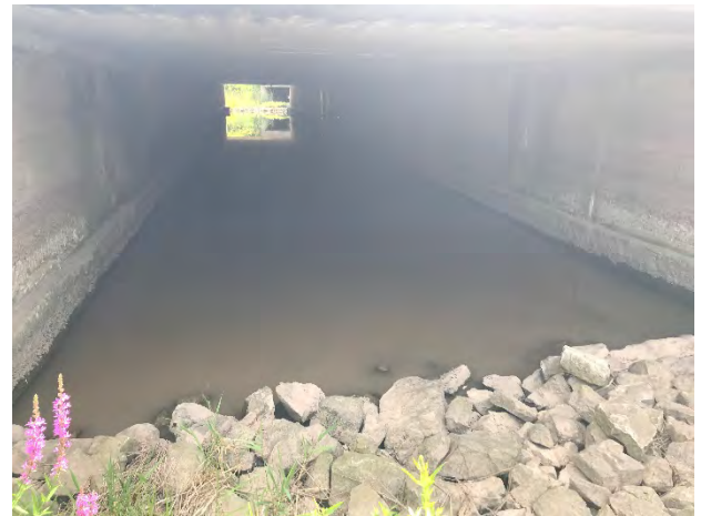
PHOTO 15 (LEFT): VIEW OF ANGULAR SCOUR PROTECTION AT QEW CULVERT INLET WHICH POSES LOW FLOW BARRIER TO FISH MIGRATION.
