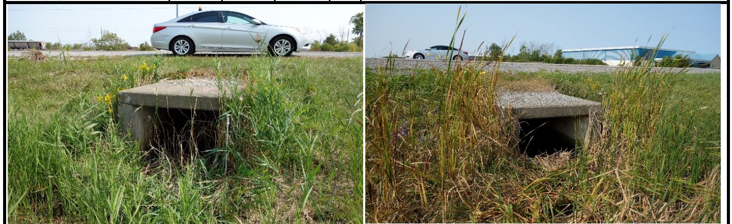
Upstream Photo Downstream Photo
