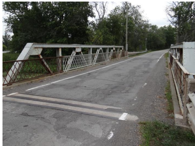
Plate 4: Oswego Creek Bridge (BHR 1), looking east.
