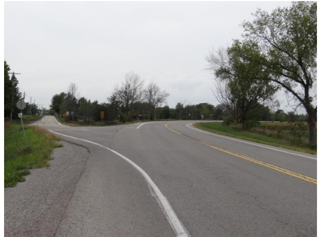
Plate 10: Intersection of Creek Road (at left) and Riverside Drive (at right), looking west.
