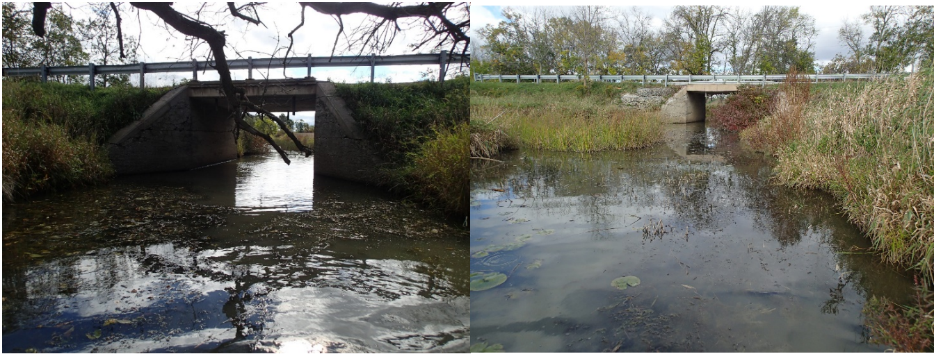
FIGURE 6 - REPRESENTATIVE PHOTOS AT CREEK ROAD BRIDGE (LEFT: UPSTREAM, RIGHT: DOWNSTREAM)
