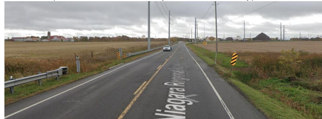
Spring Creek Tributary Box Culvert
