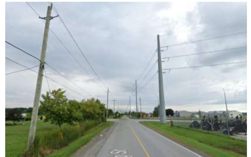
Existing hydro infrastructure
