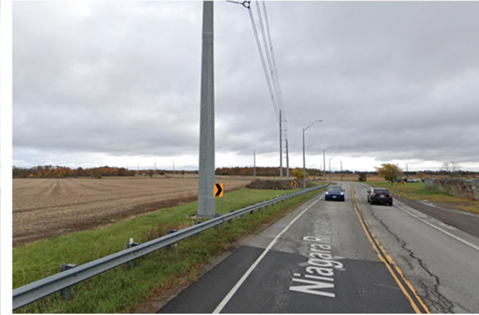
Transmission Pole adjacent to Roadway within Regional ROW along Thirty Road north of Young Street
