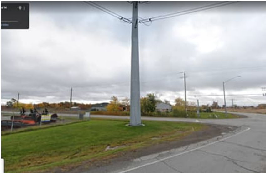
Picture 1 – Existing Transmission Pole located on Regional Property
