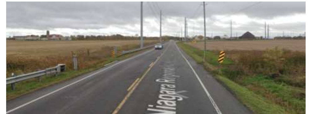
Spring Creek Tributary Box Culvert
