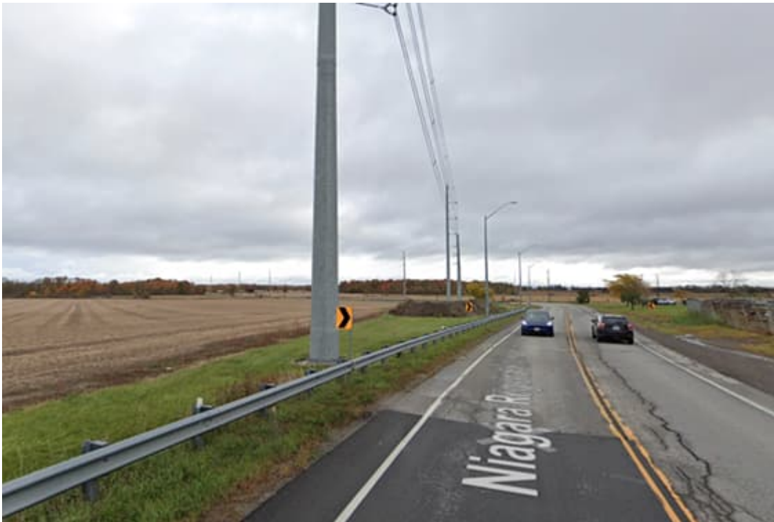
Picture 2 – Existing Transmission Pole adjacent to Roadway within Regional ROW
