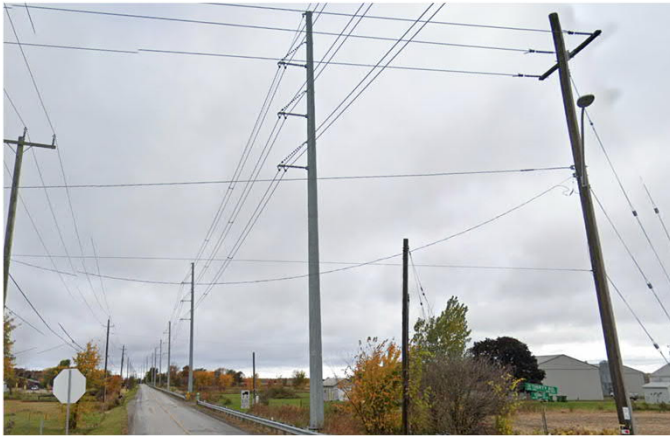
Transmission Pole adjacent to Roadway within Regional ROW (NW corner)
