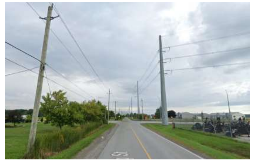
Existing hydro infrastructure
