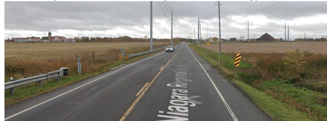
Spring Creek Tributary Box Culvert
