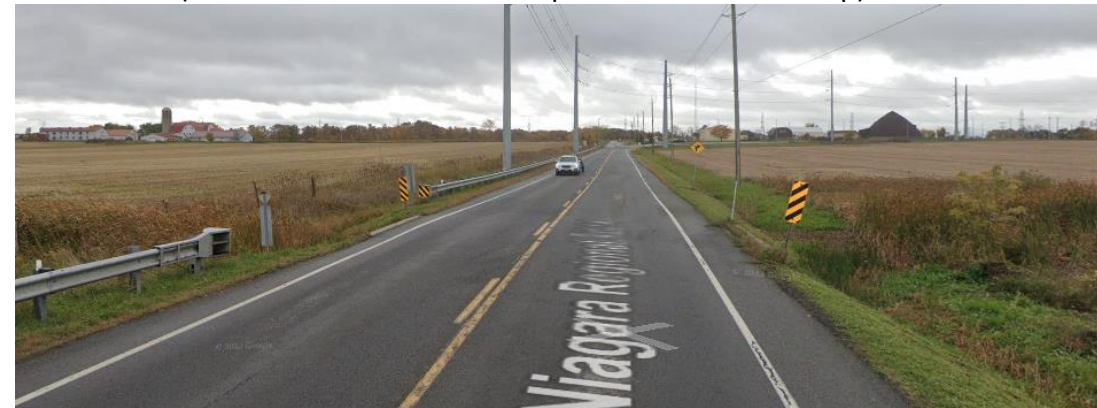
Spring Creek Tributary Box Culvert
