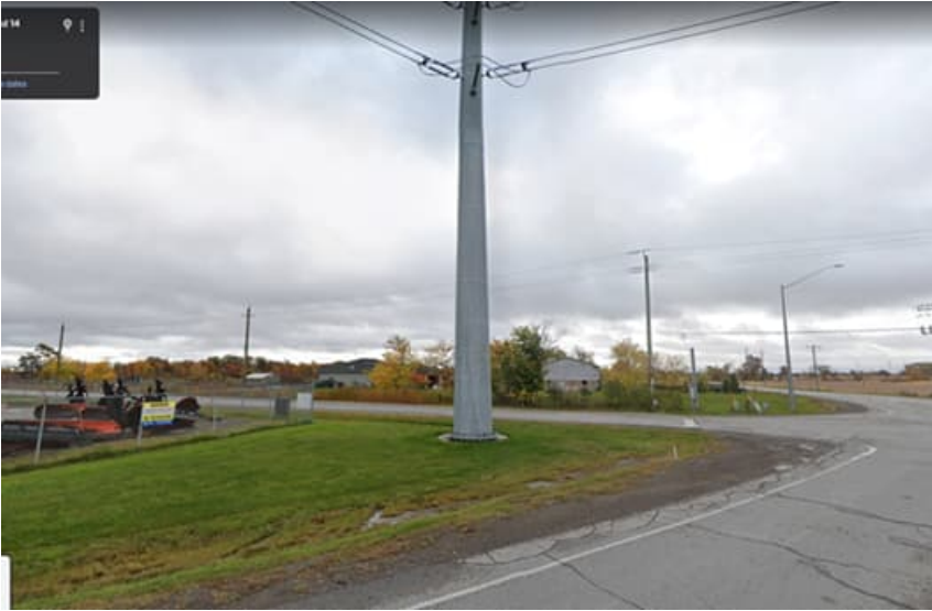
Picture 1 – Existing Hydro One Transmission Pole located on Regional Property (would be encroached upon)
