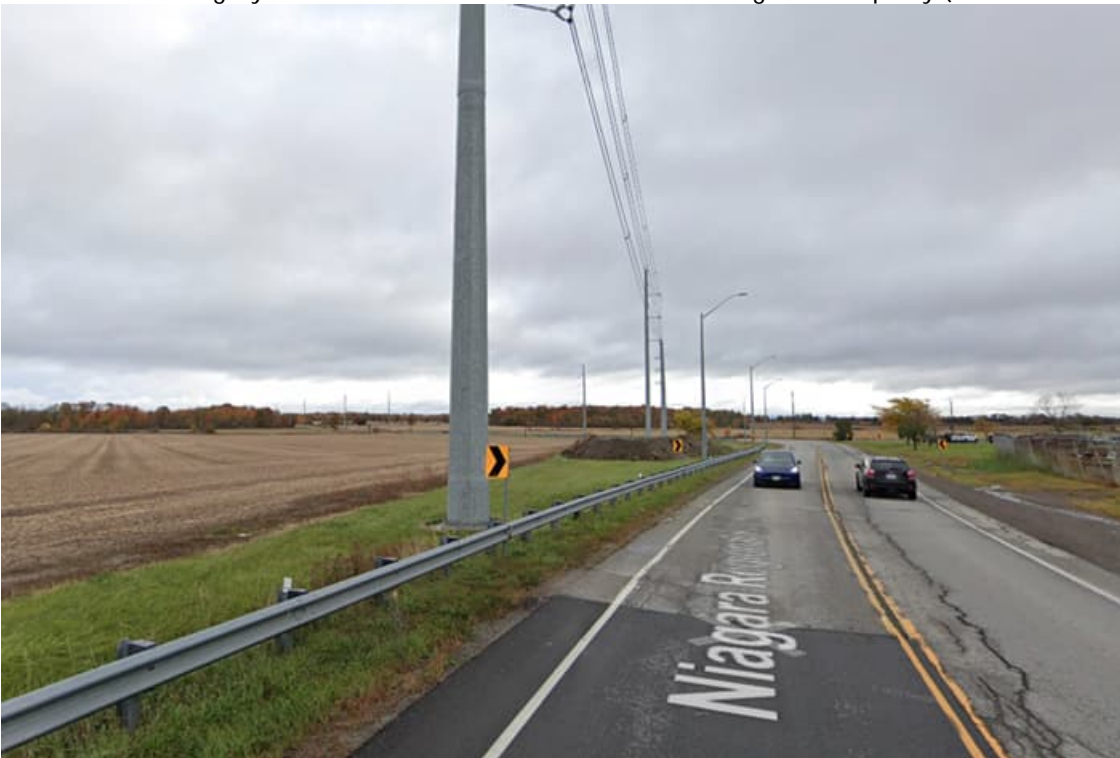
Picture 2 – Existing Hydro One Transmission Pole adjacent to Roadway within Regional ROW
