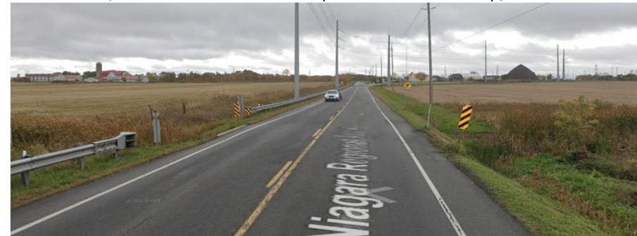
Spring Creek Tributary Box Culvert
