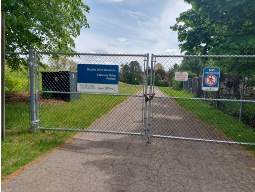
Plate 15: Entrance to Shoalts Drive Reservoir from Shoalts Drive, looking east (A.S.I., 2022).
