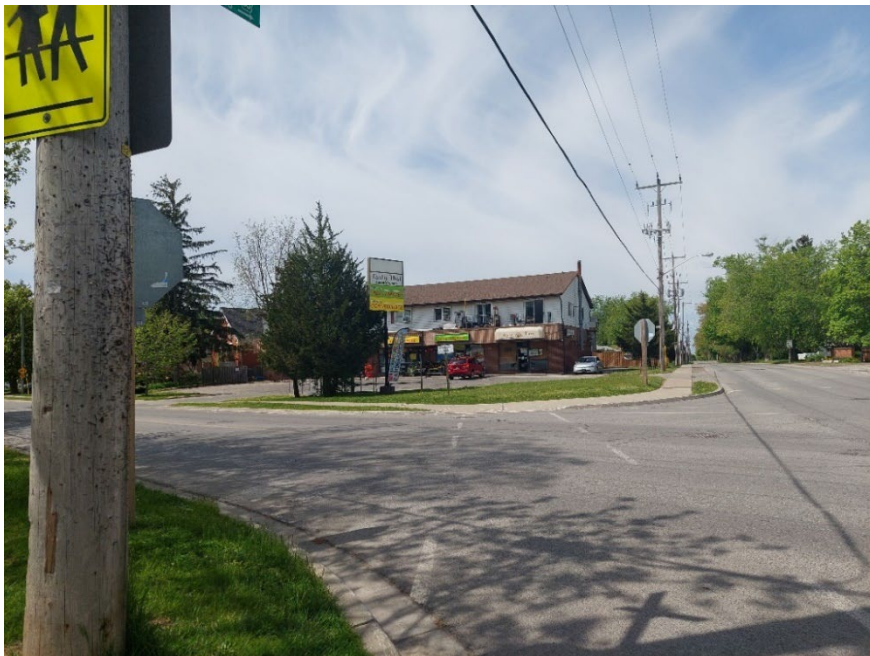
Plate 10: Commercial building on the southwest corner of the intersection of Haist Street and Canboro Road, looking west (A.S.I., 2022).
