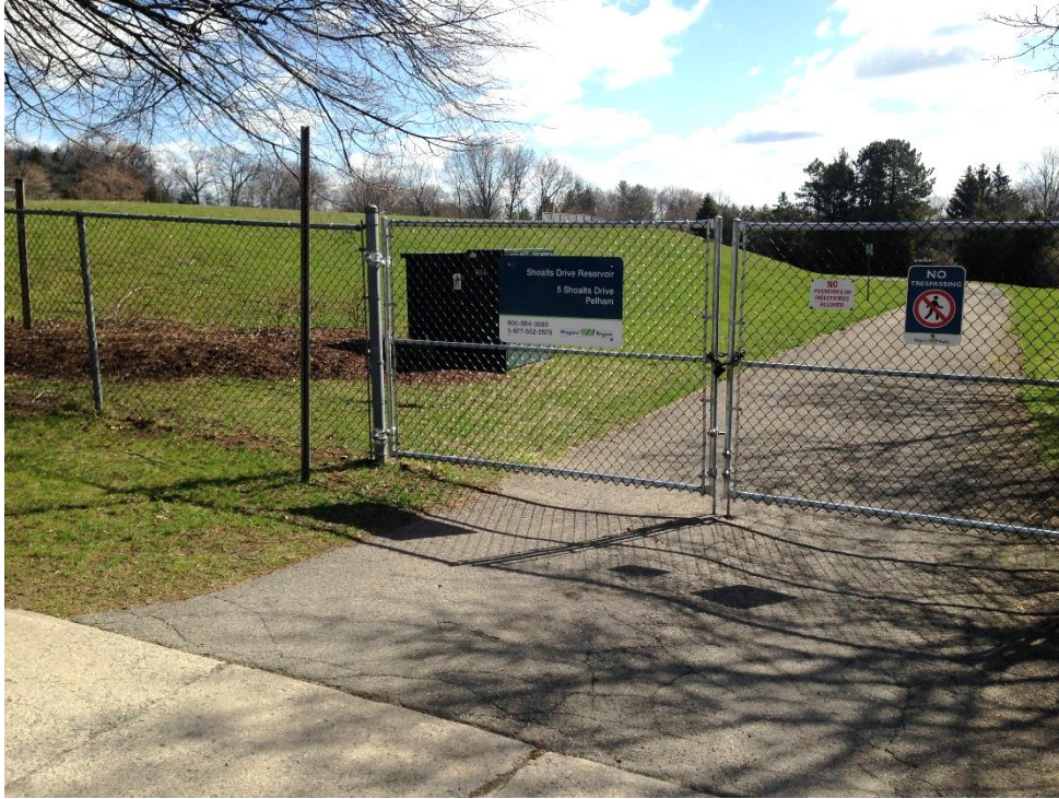
Image 15: Shoalts Drive Reservoir; previously disturbed, no potential.
