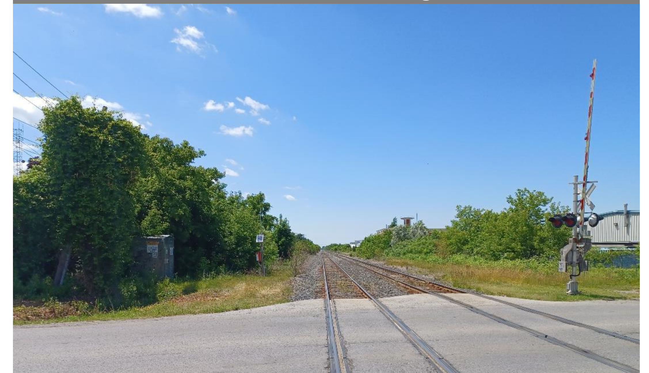
CN Rail Corridor at Louth Street, looking west
