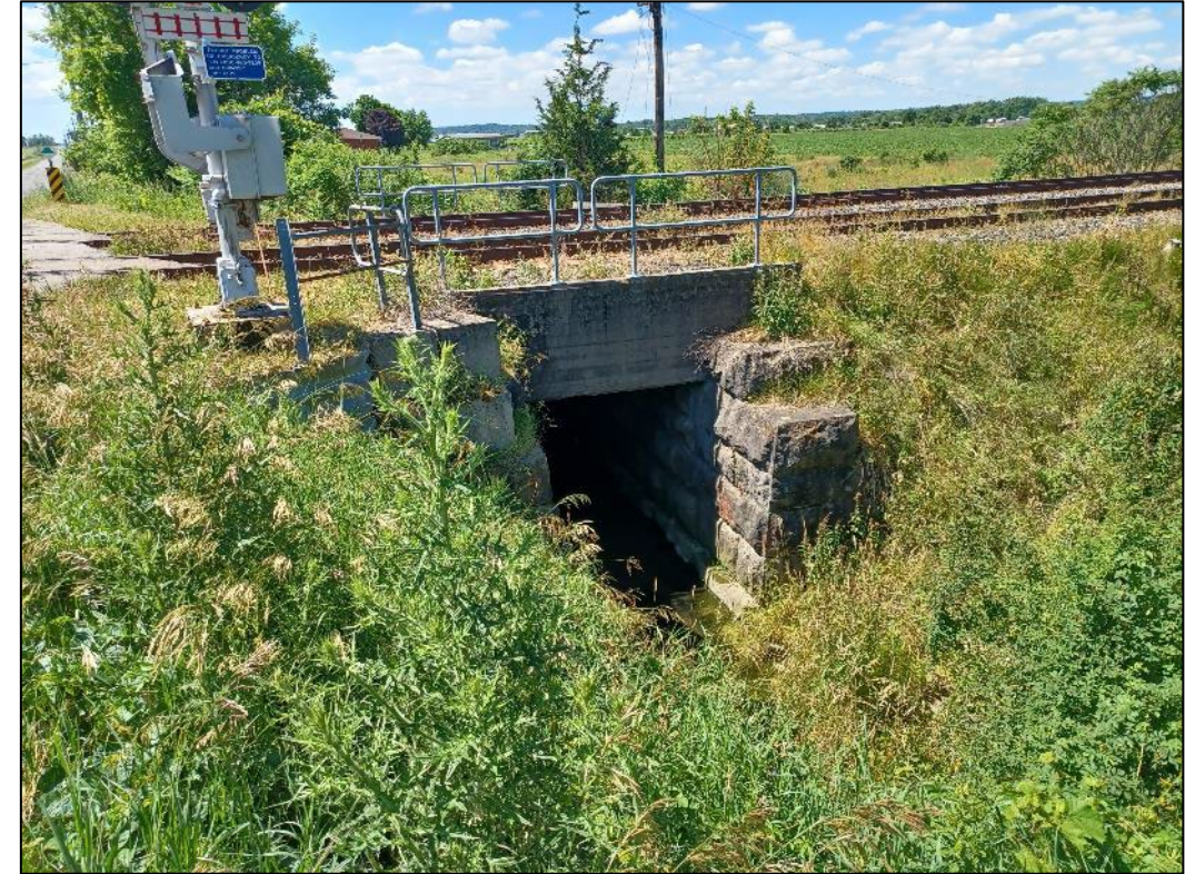
Culvert at Third Street Louth CN Rail Crossing
