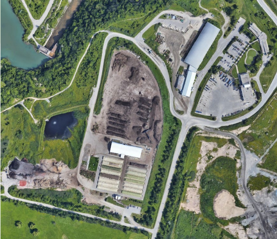
Biosolids Management Centre with Alkaline Stabilization
