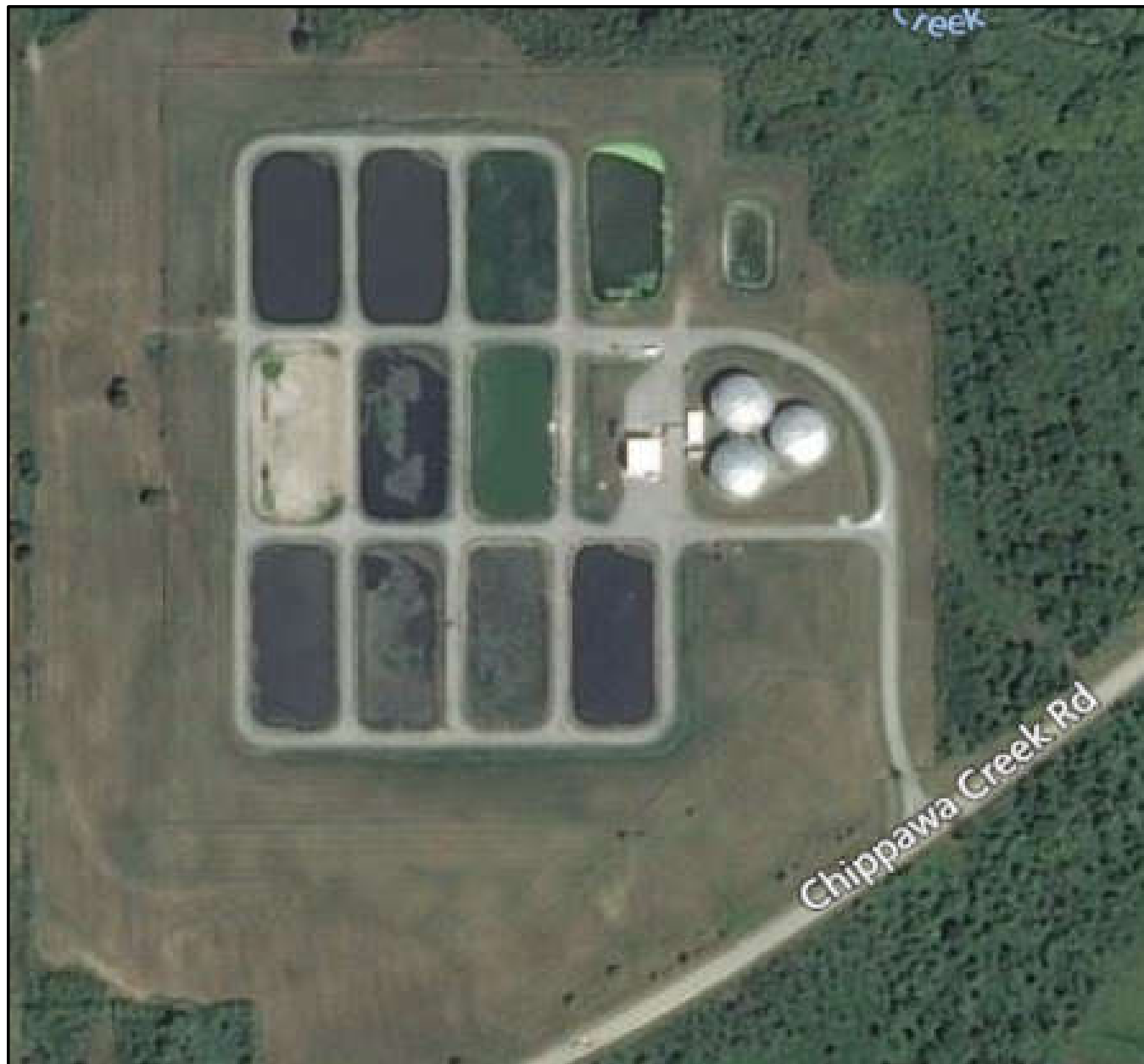
Garner Road Biosolids Facility
