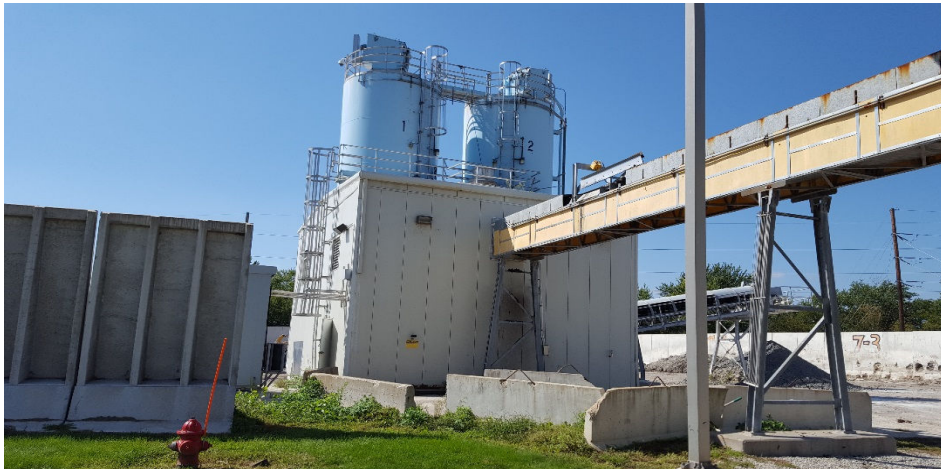
Figure 2-8 Lime Stabilization System
