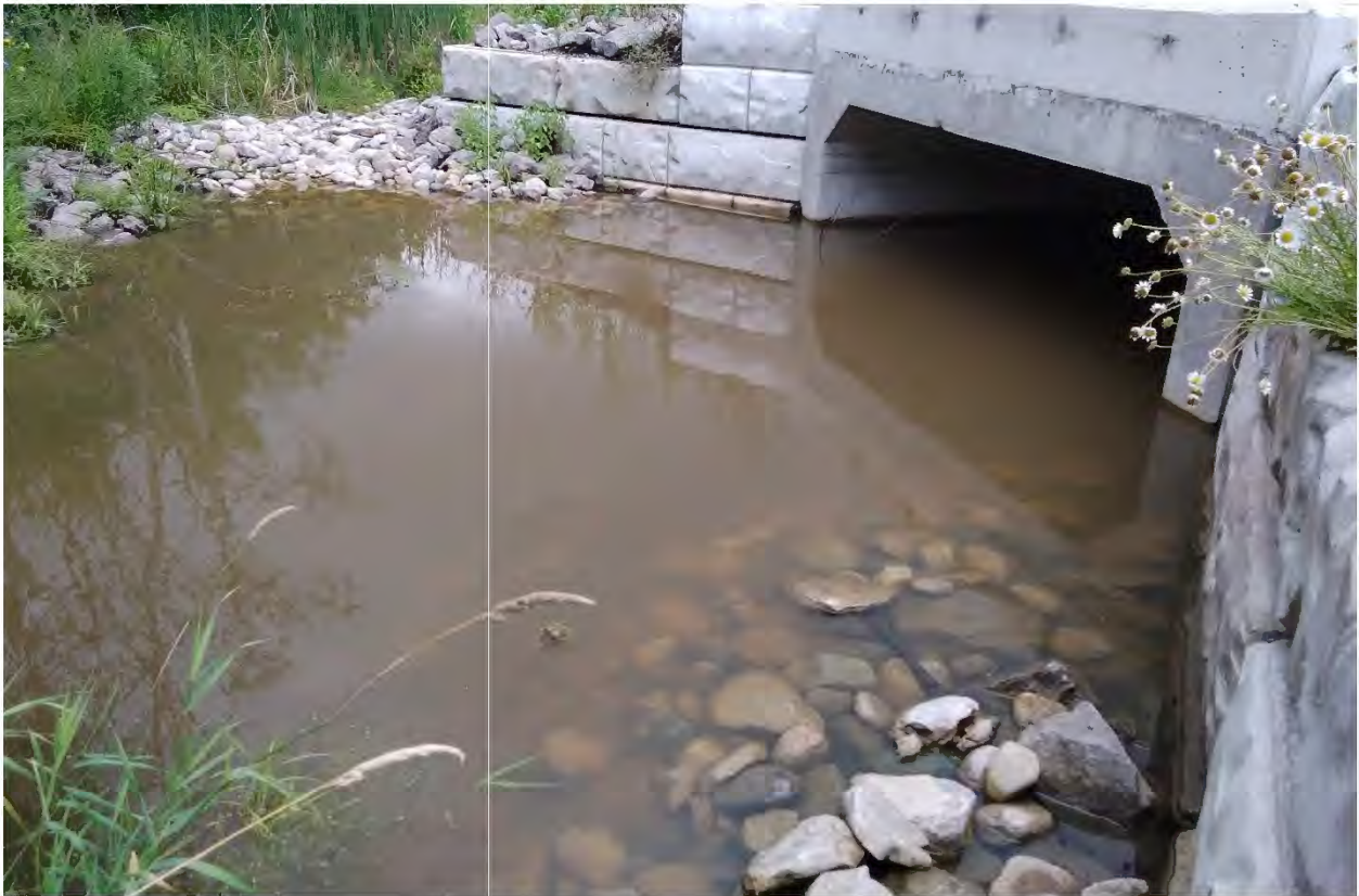
Figure 6: Culvert downstream of the Cattail Marsh
