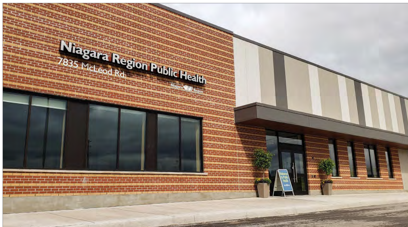
From top: ground breaking for the Niagara Regional Police Service District Facility in St. Catharines, new cell at Niagara Road 12 Waste Management Facility in West Lincoln, New Public Health and Sexual Health office in Niagara Falls.
