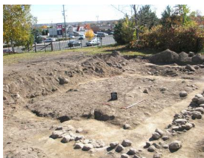
An example of a field stone foundation.
