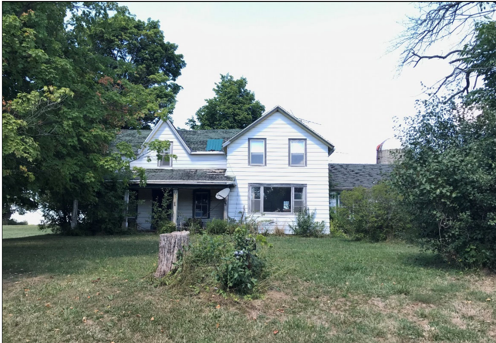
Photo 9: Residential dwelling at 6811 Reixinger Road.
