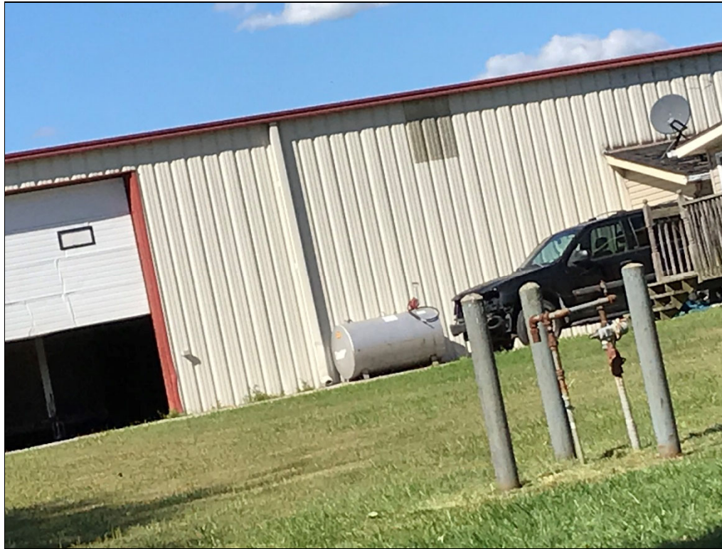
Photo 15: AST and garage/workshop at 7001 Reixinger Road.
