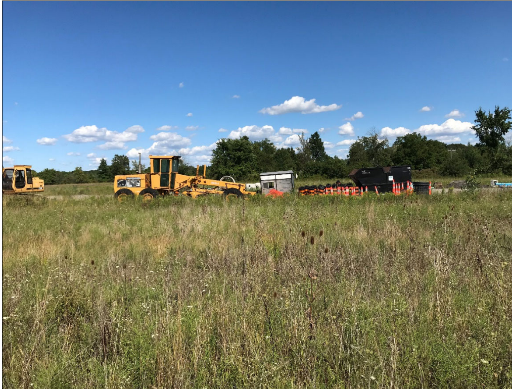
Photo 17: Construction staging area adjacent to the southern portion of the Site.
