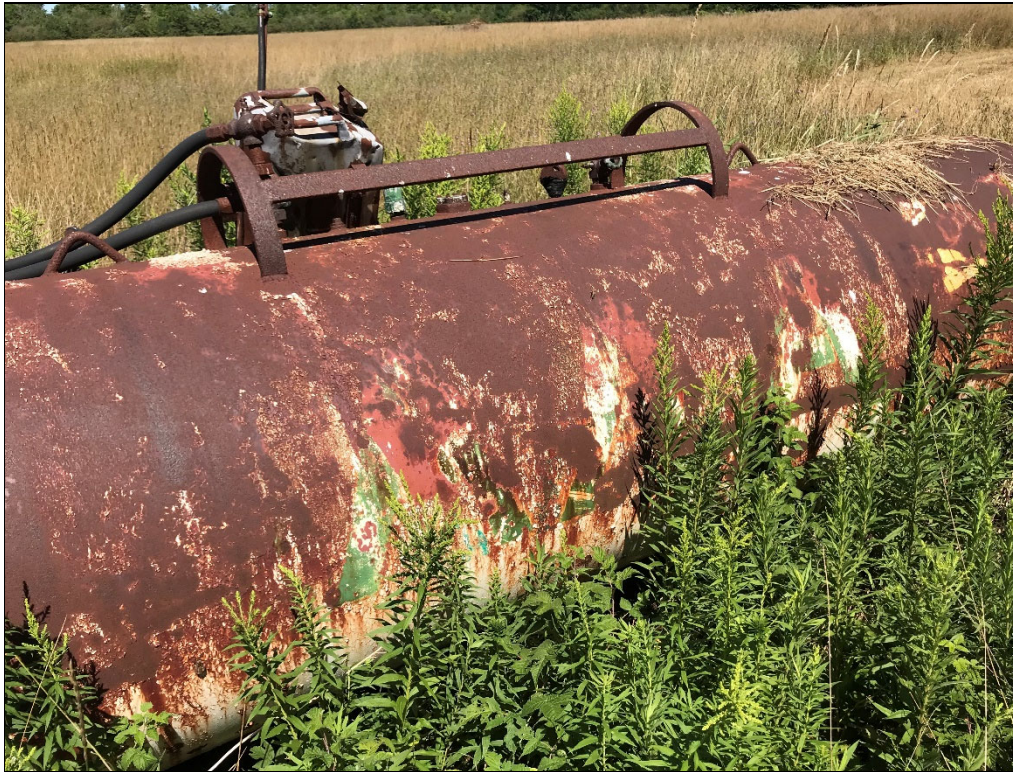
Photo 11: AST noted north of the agricultural buildings at 6811 Reixinger Road.
