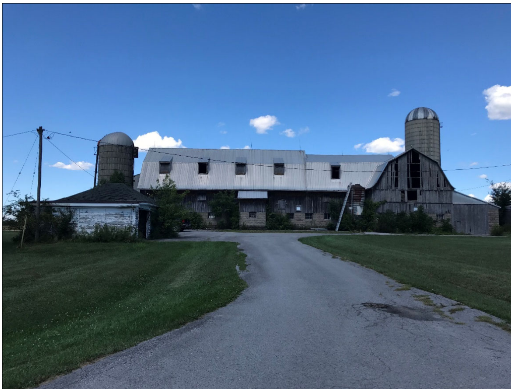
Photo 10: Agricultural buildings at 6811 Reixinger Road.
