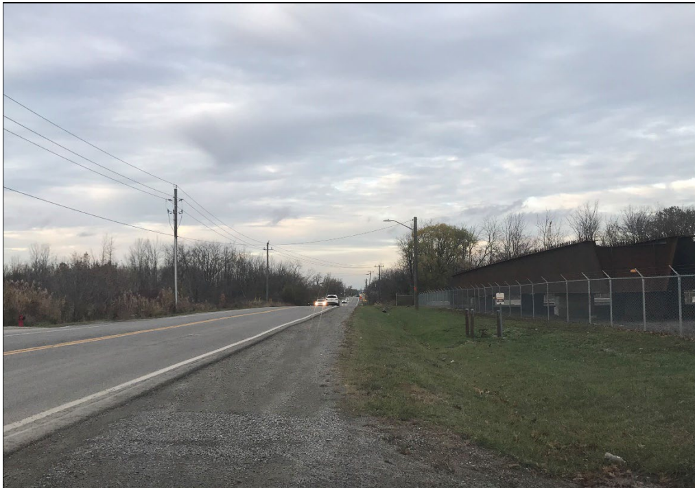
Photo 4: View of Reixinger Road from the south. Date: November 3, 2020 Direction: North
