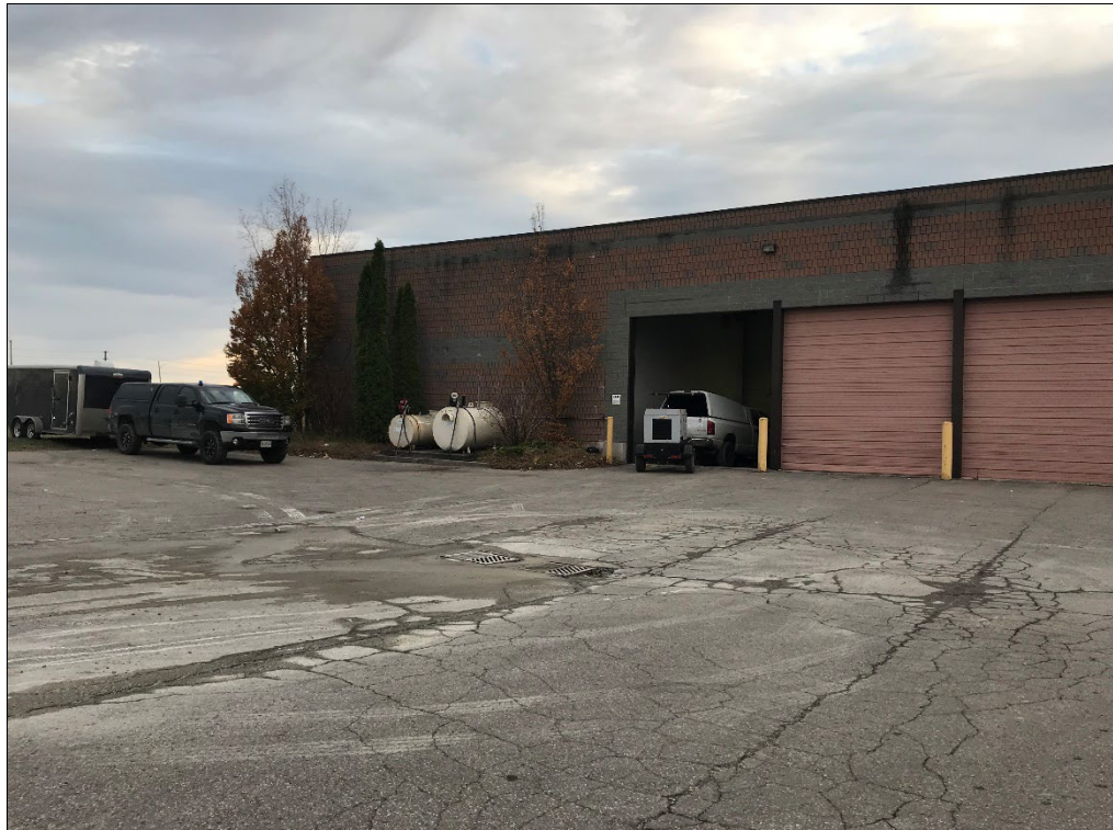
Photo 9: The two ASTs located at 7770 Canadian Drive.
