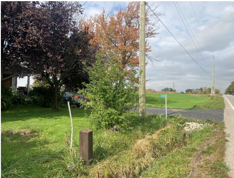
PHOTOGRAPH 12 View of the Thorold Township Road facing north. Also visible is the roadside culvert/ditching and utility box.
