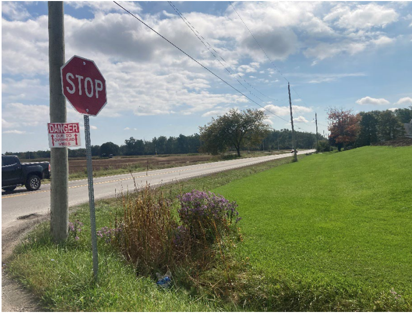
PHOTOGRAPH 11 View of the Thorold Township Road facing southeast. Also visible is the roadside culvert/ditching.
