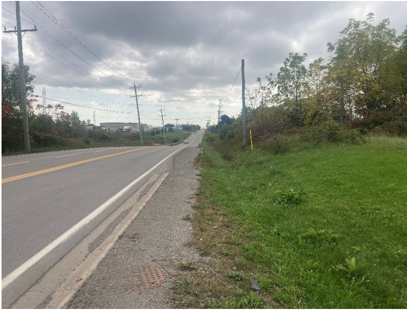
PHOTOGRAPH 5 View of Allanport Road facing south. Visible roadside culvert/ditching and manhole covering.
