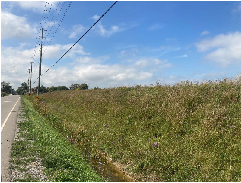
PHOTOGRAPH 7 View of Barron Road facing west. Also visible is the roadside culvert/ditching.
