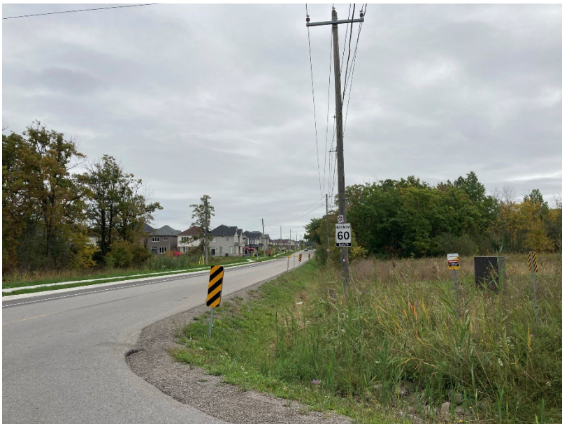
PHOTOGRAPH 32 View facing northeast of Brown Road. Deep ditching is visible on the southern side of the right-of-way.
