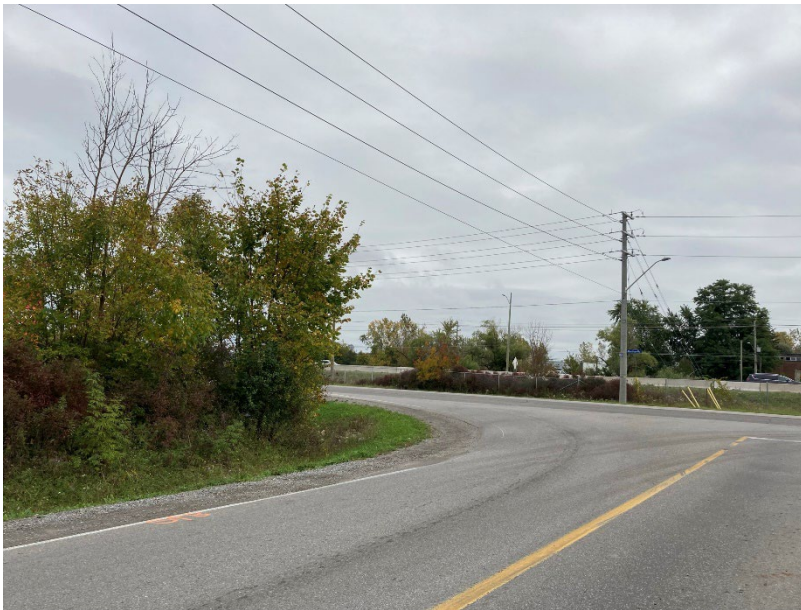
PHOTOGRAPH 36 View facing northeast of the Brown Road and Montrose Road intersection.
