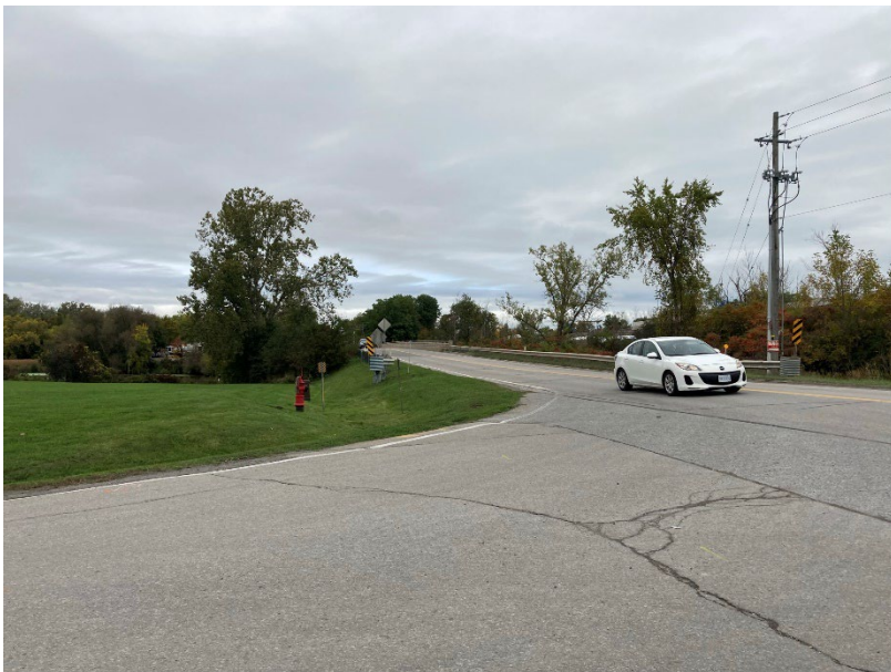
PHOTOGRAPH 22 View facing northeast toward Montrose Bridge of Montrose Road.
