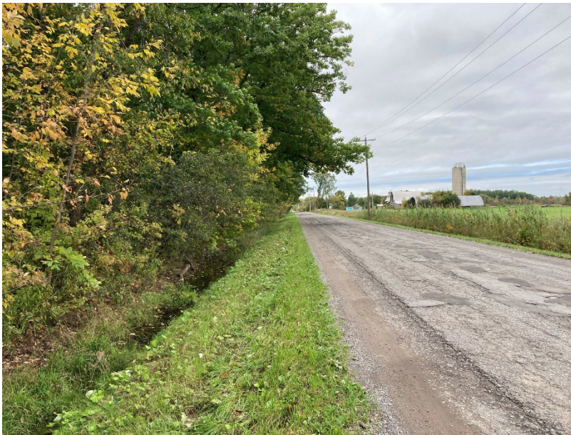
PHOTOGRAPH 2 View facing northwest toward 6811 Reixinger Road. Also visible is the deep roadside ditching.
