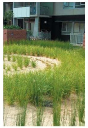
Figure: Example of bioswale incorporated within multi-unit residential development. Bioswales can be used to filter rainwater on-site.
