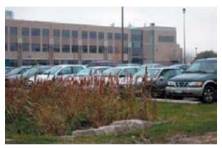
Figure: Bio Swale facilities can be incorporated into large parking areas to absorb and filter rainwater runoff.
