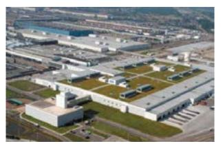
Figure: Green roofs minimize water runoff and assist building insulation systems.
