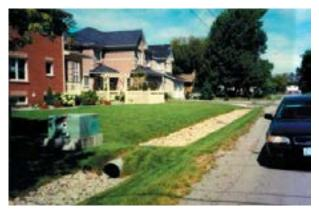
Figure: Example of swale drain in residential area. Swale drains can be used to improve rain water infiltration.
